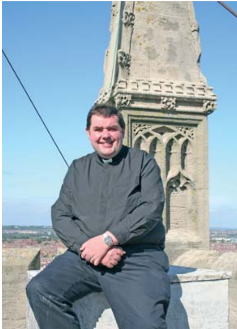
Canon Bob White at the top of St Mary's church tower. Examples of the erosion to carvings on the stonework can be seen on the pinnacle behind him. Repairs are also needed on the tower walls
