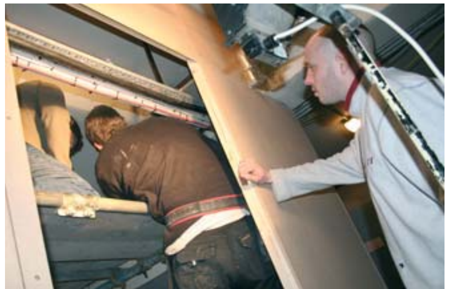
Workers from Norman Wright Construction in the cathedral cellar
